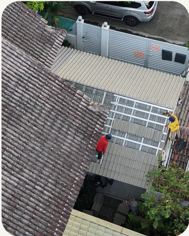
Installation: The crew at work
