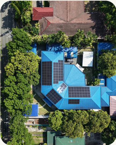
Aerial: The finished roof, from above
